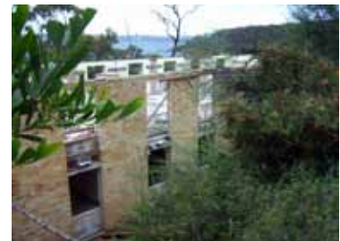
ABOVE: Building 19 - work in progress.
