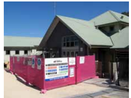
ABOVE: Building 22, now being converted to a laboratory complex.
